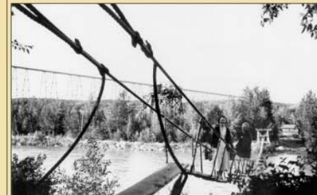
A cable 'swinging' bridge allowed mine workers to cross the river near the mine, instead of making the long trip by road. A portion of the tippie can be seen in the distance.
